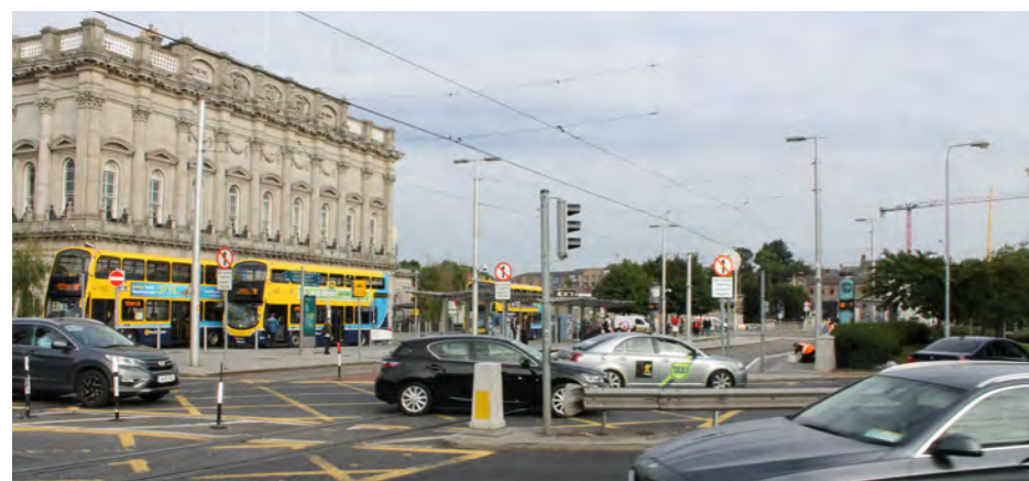
Heuston Station - St. John's Road
