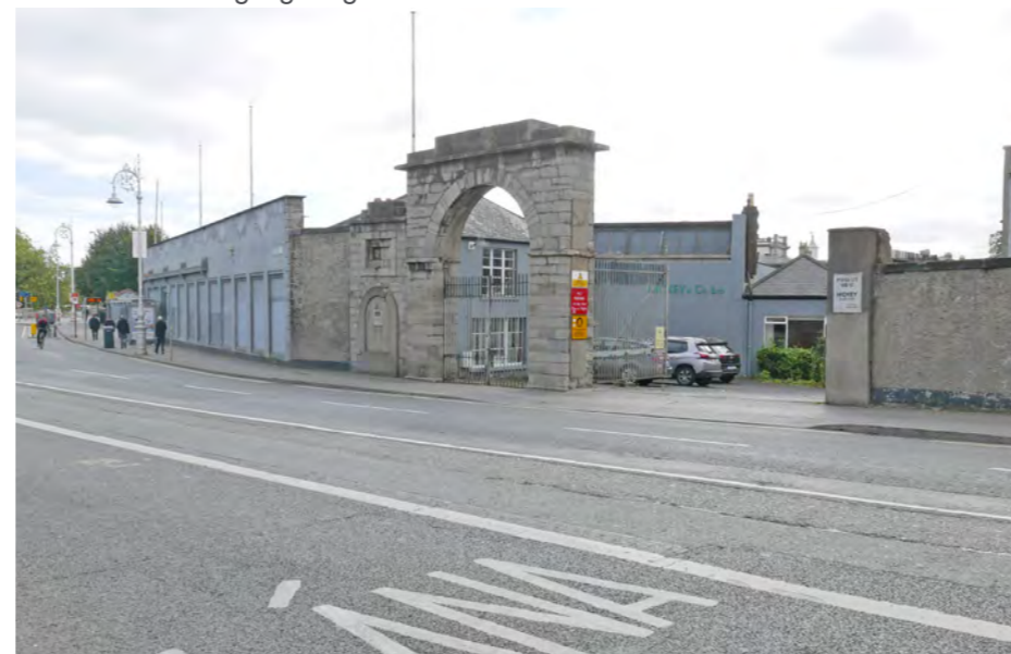
Parkgate Street - Existing Stone Arch
