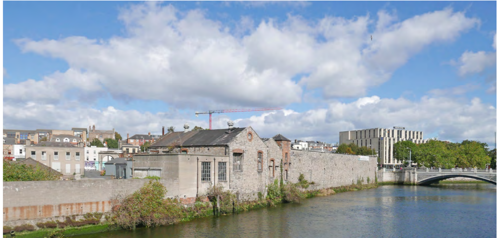
View of Existing River Wall towards Sean Heuston Bridge
